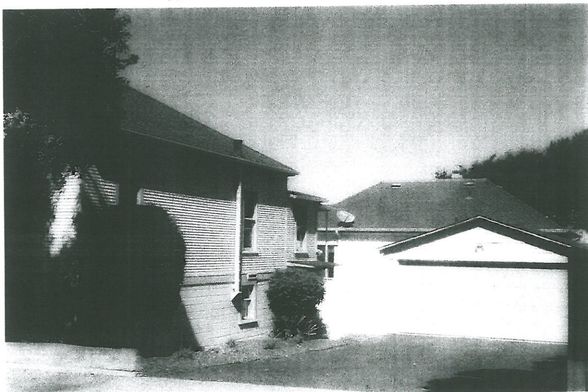
Photo #2. Looking NW at the east side-elevation & detached modern garage, Kent Seavey, October 8, 2016.
