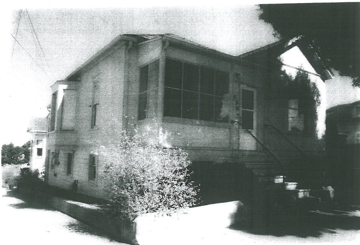
Photo #3. Looking NE at the south facing façade & west side-elevation, note The later enclosed porch, modern door, staircase & metal railing Kent Seavey, October 8, 2016.
