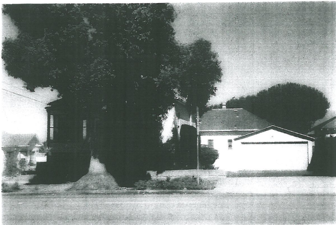
Photo #1. Looking north at the south facing façade & detached modern garage, Kent Seavey, October 8, 2016.
